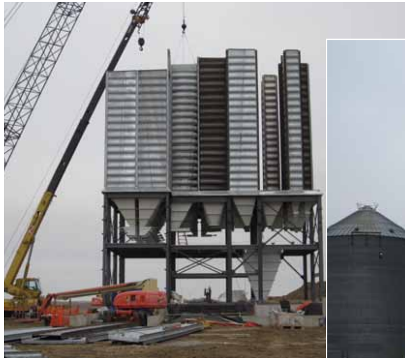
The StateLine Cooperative Halfa Feed Mill now has a completed grain leg, which has a 20,000 bushel per hour receiving capacity. Construction on the 600,000-bushel bin will begin in spring.
