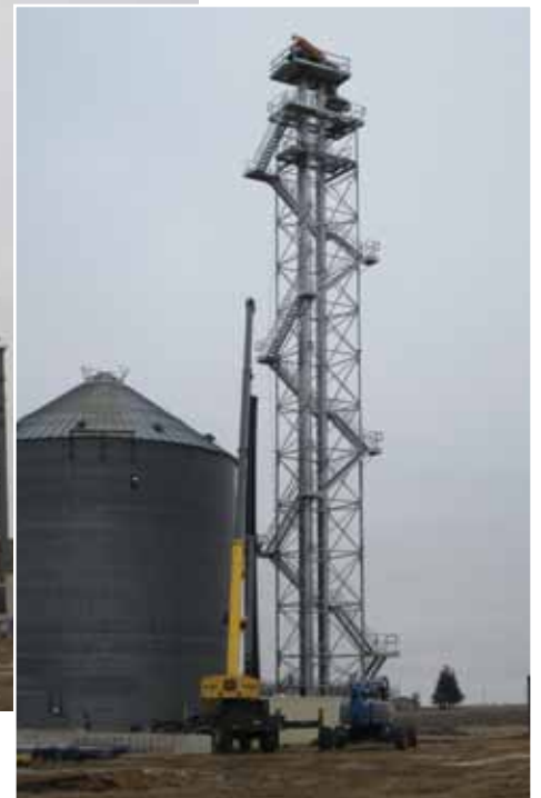
The StateLine Cooperative Halfa Feed Mill now has a completed grain leg, which has a 20,000 bushel per hour receiving capacity. Construction on the 600,000-bushel bin will begin in spring.
