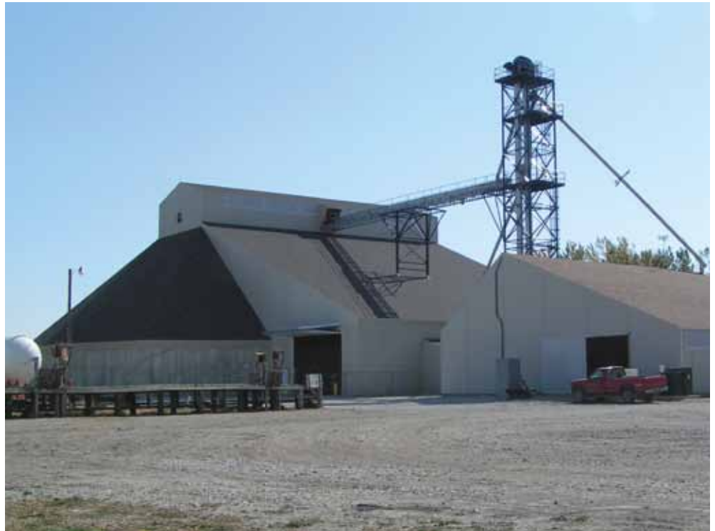
StateLine Cooperative's Armstrong fertilizer storage was completed in 2011.
