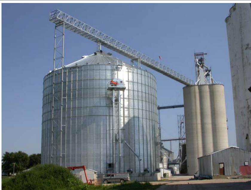
Electrical work is being finalized now on Rippey's new 680,000 bushel bin.
