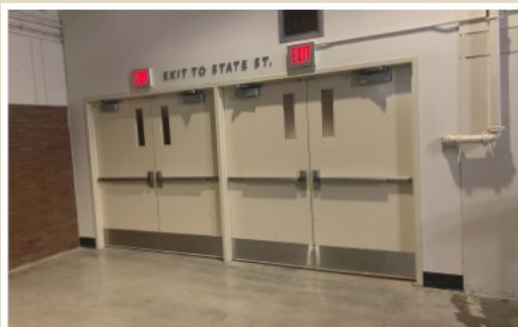
2nd floor doorway leading to Stairwell 7
