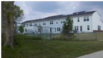
Needs weeded at fence line
