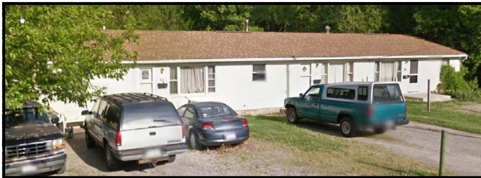
413-417 North Granville Street, Baltimore, Ohio
