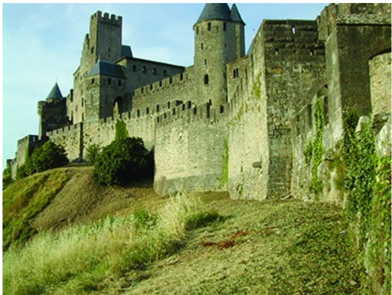
One of the most beautifully preserved medieval walled cities is Carcassonne, France. Notice the use of a double wall.
