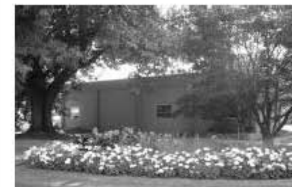
CBWMP Operations Center (LEED registered project), City of Portland, OR
