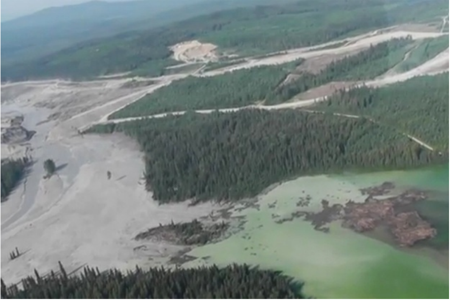
The former Mount Polley tailings dam. (via www.vancouverobserver.com )
