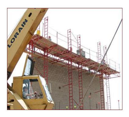
New requirement to address climbing of end frames, OSHA allows climbing up to 34 feet w/out fall protection
