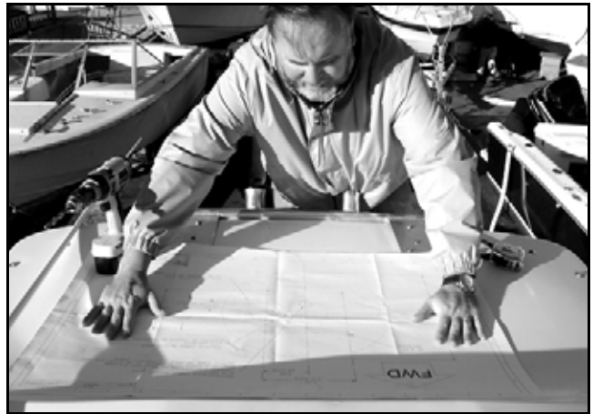
Figure 6: Using the Template to Mark Hole Locations
