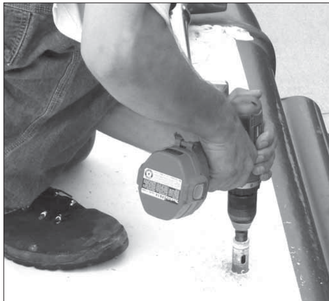
Figure 11: Drilling the Cable Access Hole
