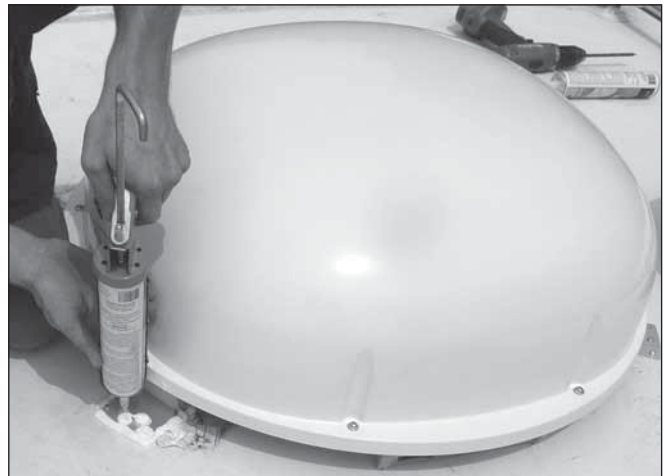
Figure 9: Sealing the Fasteners
