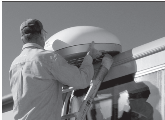
Figure 5 Carrying Antenna to Roof
