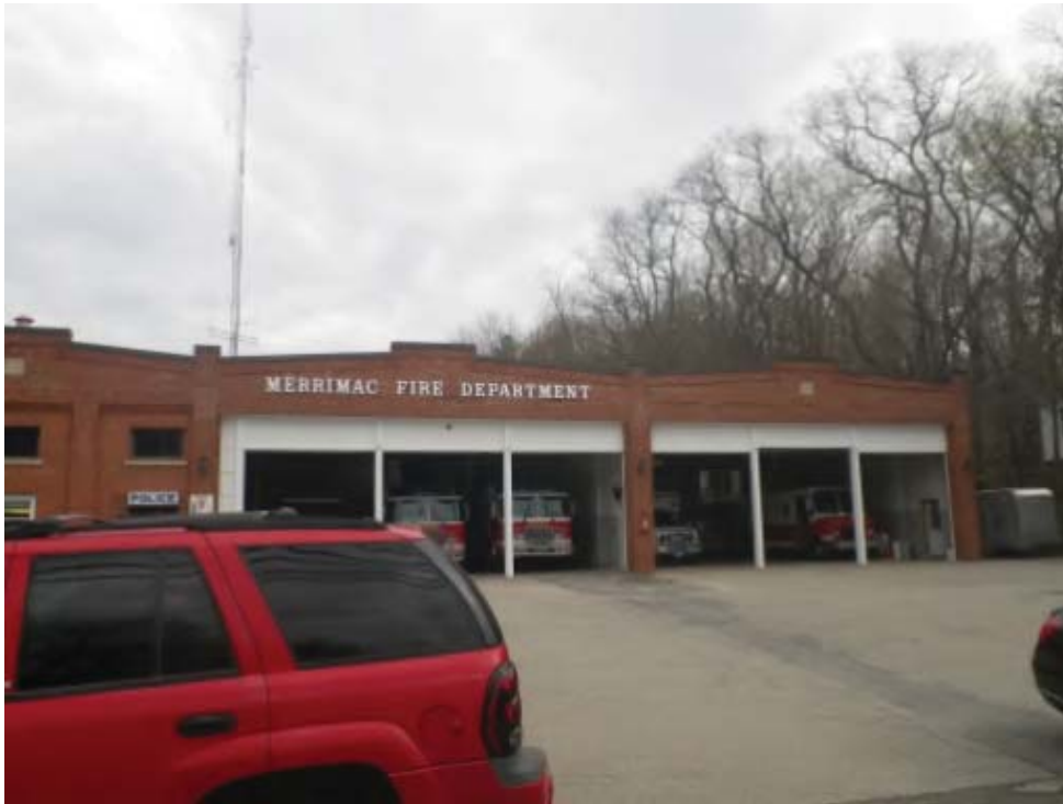
Photo 01 - Southern Elevation of Building
