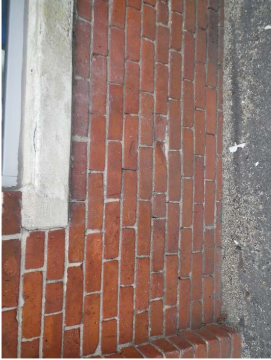
Typical exterior brick masonry wall
