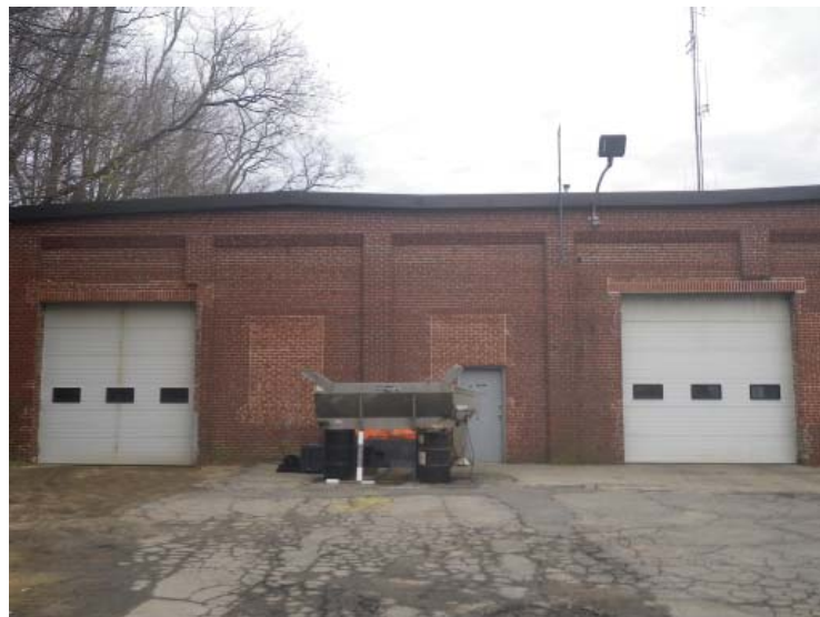
NORTH WALL: OVERHEAD DOORS AT PUBLIC WORKS.
