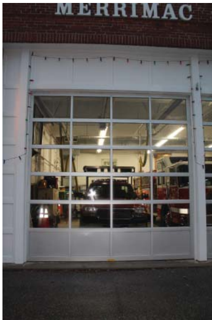
OVERHEAD DOOR AT FIRE DEPARTMENT
