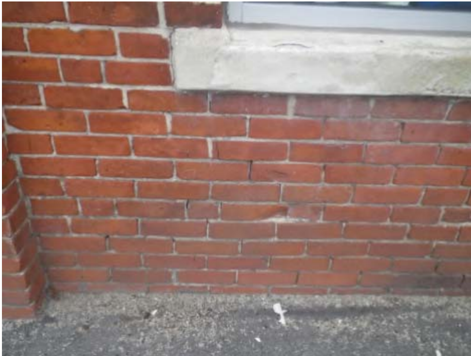
Photo 05 - Typ brick condition
