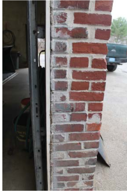
BRICK PIER AT OVERHEAD DOOR.
