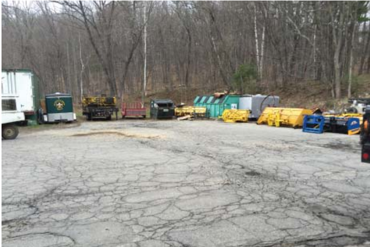
REAR OF SITE LOOKING AT PUBLIC WORKS YARD + EQUIPMENT.
