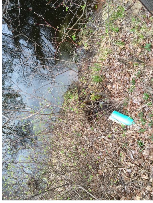
Basement pump pipe outlet
