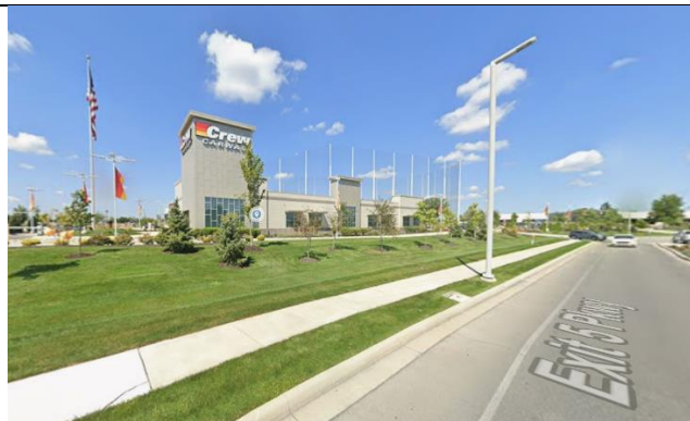
Crew Carwash – Fishers, Indiana (Built 2020)
