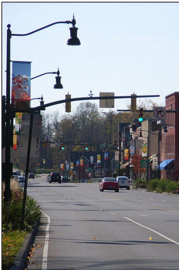
U.S. 40 is classified as a major arterial roadway
