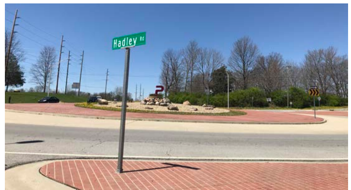
Roundabout improvements at Hadley and Center Streets. Source: HWC Engineering
