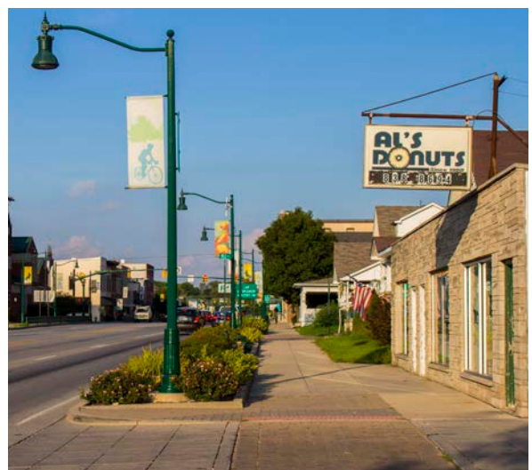
Downtown Plainfield Streetscape Source: HWC Engineering
