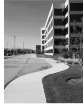
Pull-Off Loading Area
