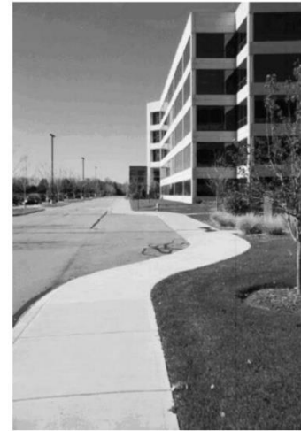
Pull-Off Loading Area
