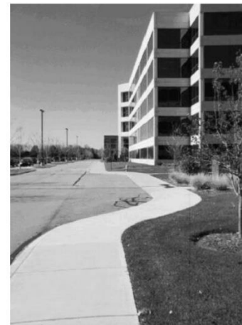
Pull-Off Loading Area
