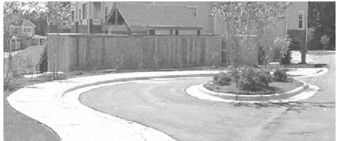
Vehicular pull-off at Refuse/Reuse Container Enclosures
