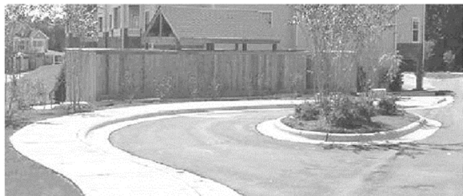
Vehicular pull-off at Refuse/Reuse Container Enclosures
