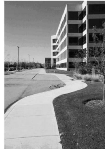
Pull-Off Loading Area
