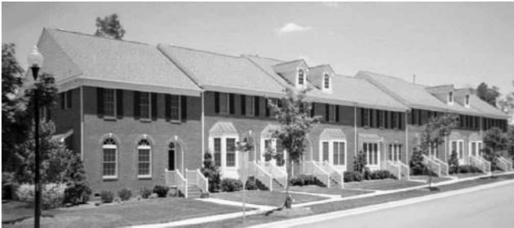
Multi-Family Townhouses with Roof Lines Changes
