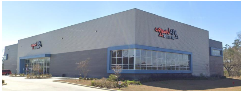
Figure 2: Denham Springs, Louisiana
