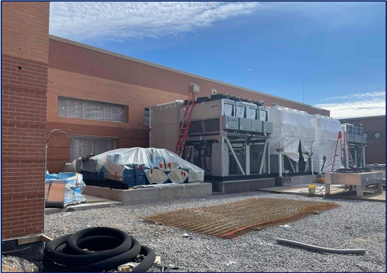
AHU Installation (Under Construction) in Nashville, TN
