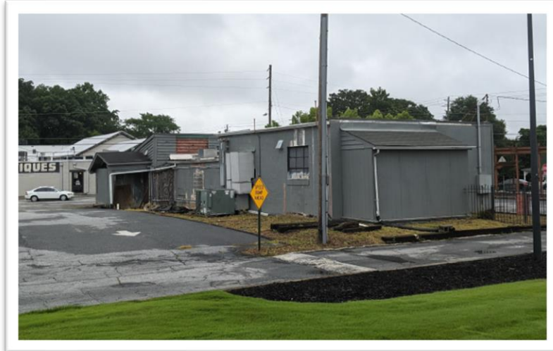
View of the rear side of the building from City Hall.
