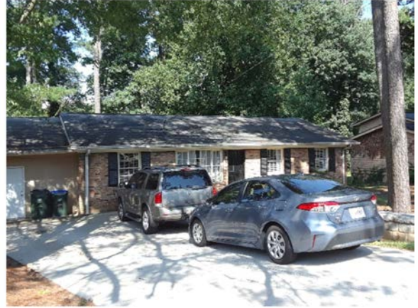
3731 Chamblee Dunwoody Rd
