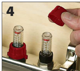
4 Flow meters and memory stops are built in
