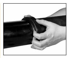
**ALIGNMENT**— After aligning the two pipe ends together, pull the gasket into position, centering it between the grooves on each pipe. The gasket should not extend into the groove on either pipe.
