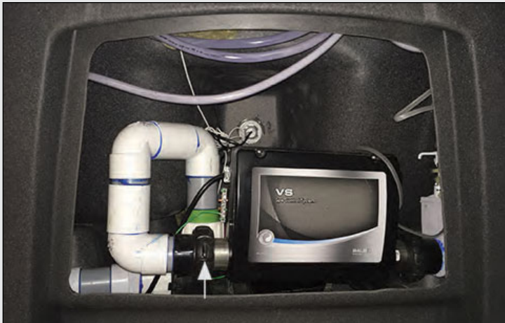
FIGURE 1.2a : HEATER UNION; LOOSEN UP TO BLEED AIR
