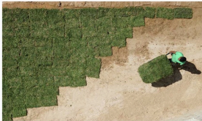
A man wheels pallets of sod between homes in a newly built neighborhood in Conroe Houston Chronicle Staff
