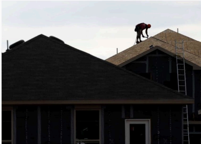
A man works on framing a roof on a home in a subdivision near Texas 242 and F.M. 1314 Houston Chronicle Staff
