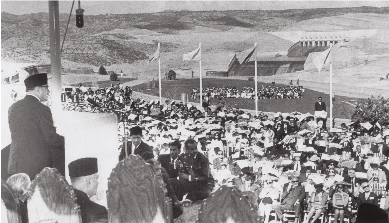
President Ayub Khan addressing a ceremony held to mark the inauguration of the Mangla Dam project along the banks of the Jhelum River in 1967. The Dam was an important component of the Indus Waters Treaty. | Photo: The Tahir Ayub Collection
