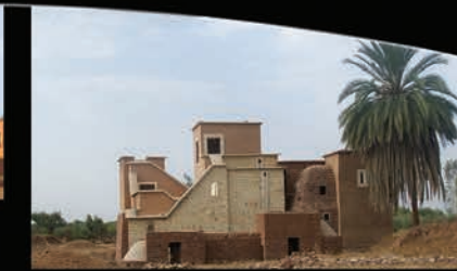
Housing rehabilitation in Morocco, Algeria and Tunisia, in collaboration with the Arch. Taj project in Marrakech. (Presented at COP 22)
