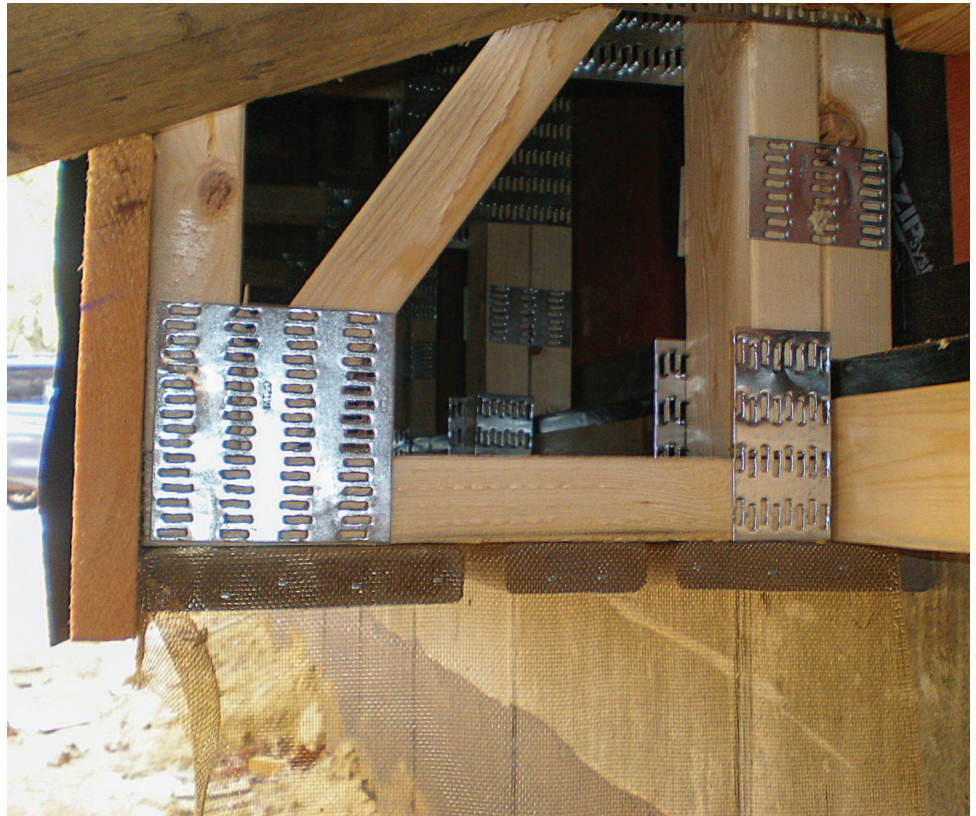
BUTTON UP THE BOTTOM Larsen trusses sometimes sit atop the foundation or the foundation insulation, and sometimes hang outside of the foundation. In any case, you'll need to be able to keep insulation in and critters out. On this project, a combination of insect screen and synthetic deck boards get the job done.
