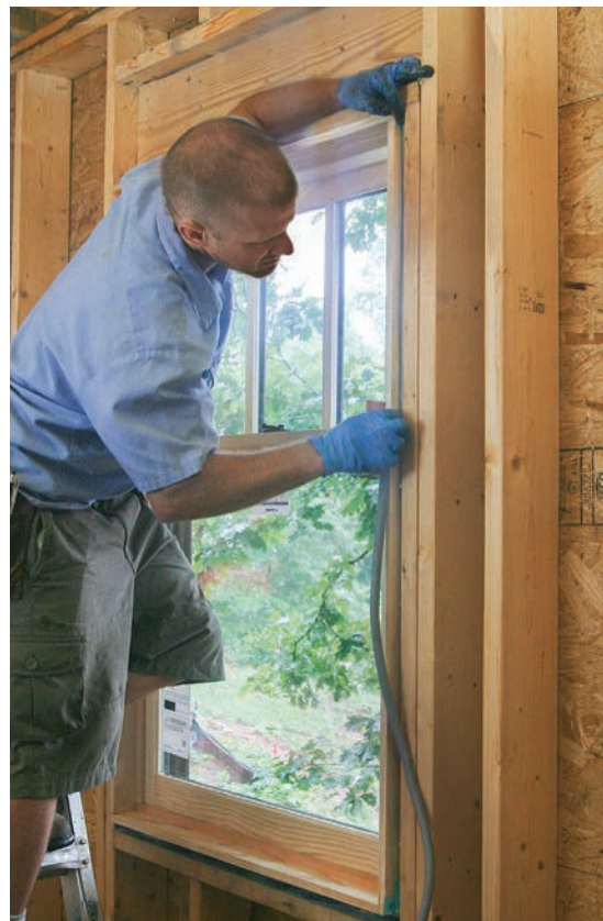
A caulk joint that will last. Foam backer rod cut and pressed in around the window jamb creates a flexible base for the bead of caulk that follows it. Use a wet finger to smooth the bead against the backer rod, creating the ideal hour-glass shape that allows the sealant to expand and contract without cracking or debonding.
