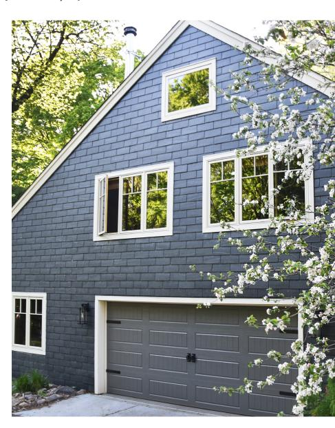
and the materials freezes and thaws without damage. When used as siding, only extreme catastrophic weather or malicious acts of vandalism might damage the tiles.
