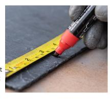
locations for the two new screw holes you need to add on the edge opposite from the predrilled ones. Mark the holes 3/4 inches away from the bottom edge and 3 inches from the left and right edges of the tile. Use a 1/4-inch masonry bit to drill two holes.
