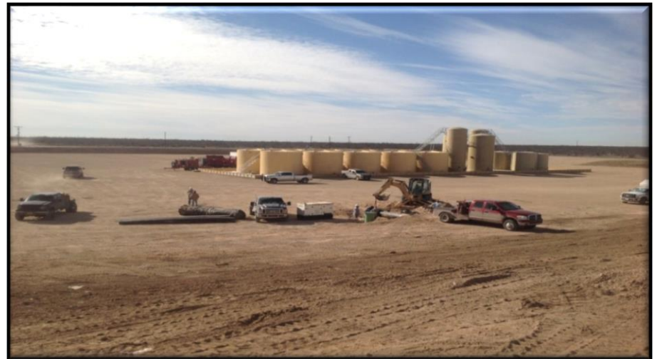
Water Recycle Facility (Under Construction)
