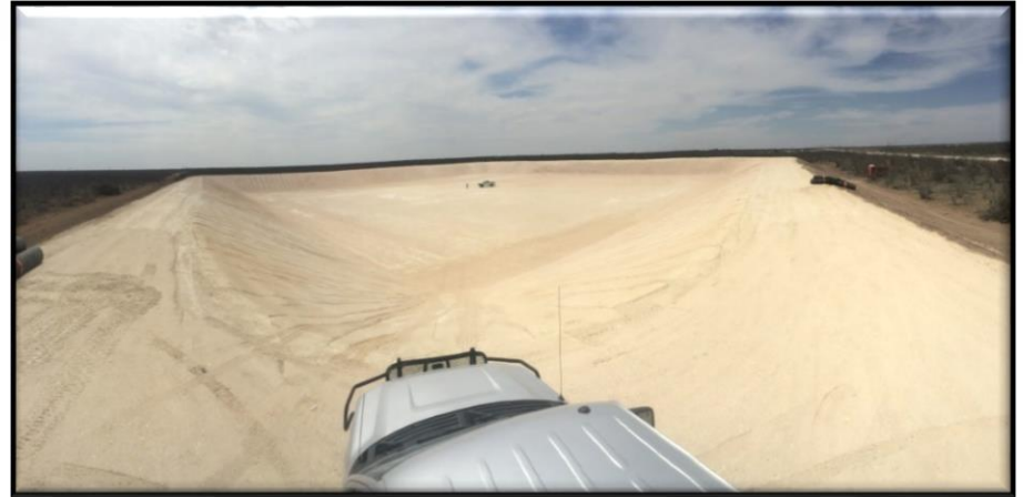
Reagan North Corridor 800,000 Bbl of Water Pit
