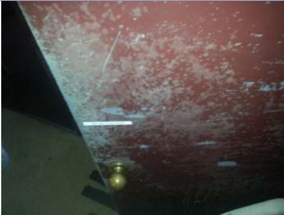
PICTURE 11: THE WHITE DISCOLORATION IS FUNGAL GROWTH ON AN FIRST FLOOR DOOR.
