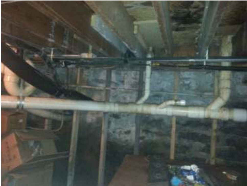
PICTURE 2: ONE OF SEVERAL BASEMENT ROOMS.
