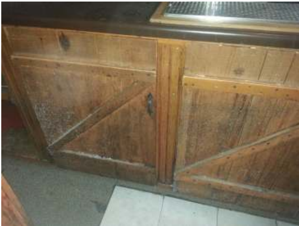
PICTURE 10: THE WHITE SPECKLING IS FUNGAL GROWTH ON THE CABINET DOORS BELOW THE BAR.
