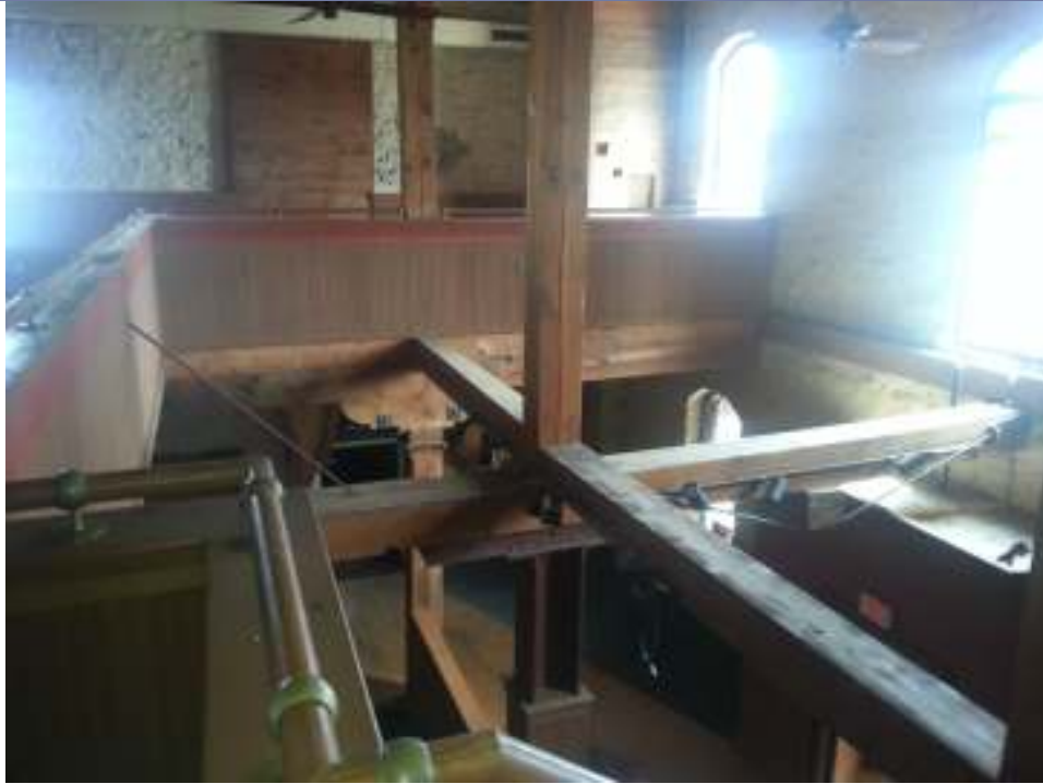
PICTURE 17: DECORATIVE BEAMS BETWEEN THE FIRST AND SECOND FLOORS.
