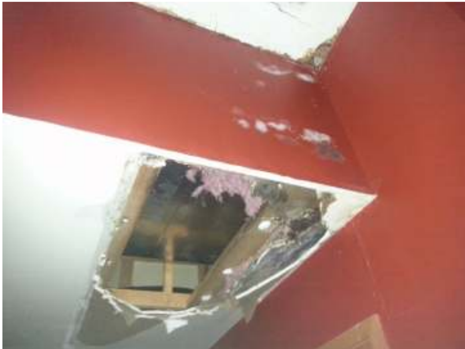
PICTURE 16: CLOSE-UP OF CEILING SHOWN IN PREVIOUS PICTURE.
