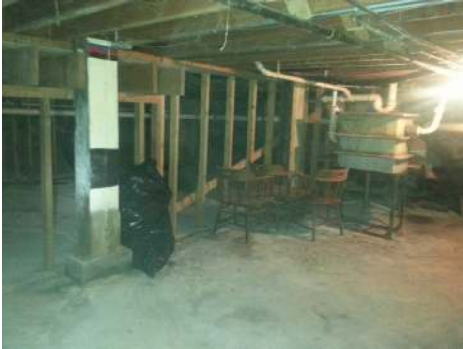
PICTURE 1: OVER OF SEVERAL BASEMENT ROOMS.
