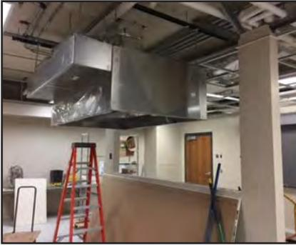
Grease hood and duct work have been installed (above).
