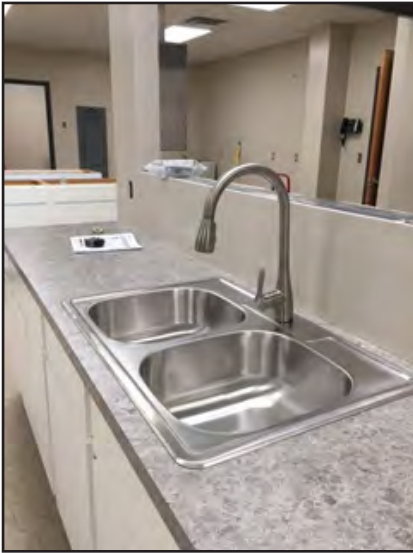
New laminate countertops and new sink.
