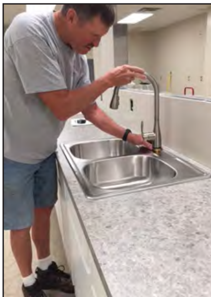
Brad Southwick installing sink and faucets.
