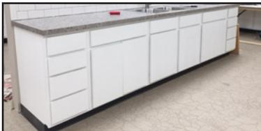
**Drawers** are installed. They are made of solid maple, have dovetailed corners, and are good quality.
