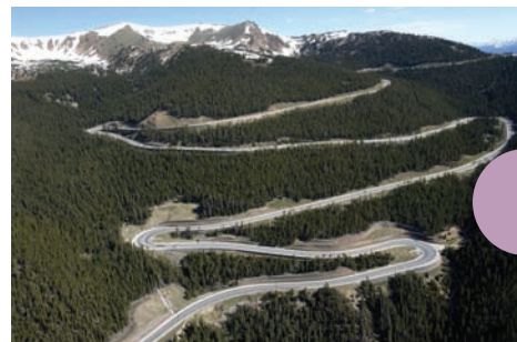
Figure 5.23 By decreasing the slope of the road, the car travels a greater distance but with less required force.
