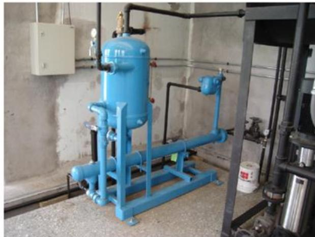
**Figure 3. Example of an integrated blowdown separator, courtesy of Wilson Engineering.**
