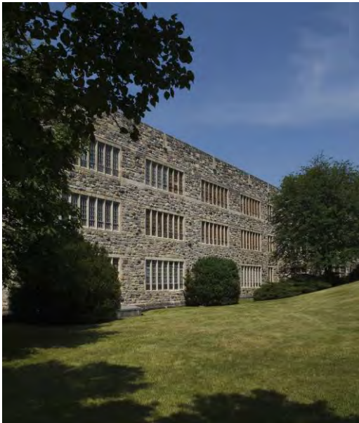
Figure 10. Norris Hall Classroom Windows, Grassy Side
