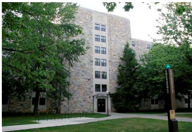
Figure 3. Exterior of West Ambler Johnston
