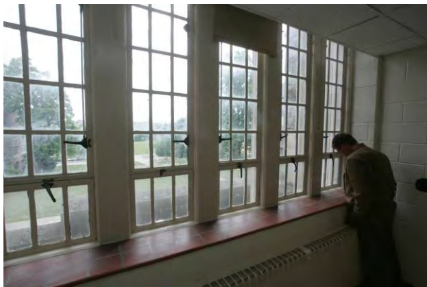
Figure 11. Typical Set of Windows in Norris Hall
