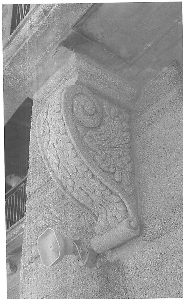
Figure 8. Replacement precast concrete bracket that was installed below the balcony (WJE)
