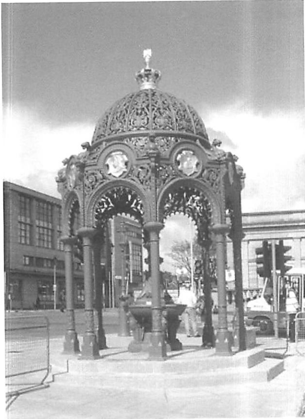
Figure 5. Dun Laoghaire Fountain Canopy, Dublin (Heritage Engineering, Glasgow)
