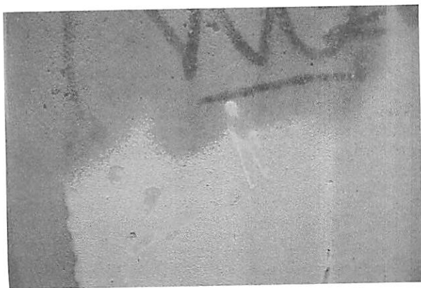
Figure 7. Use of a chemical poultice to remove graffiti. (WJE)
