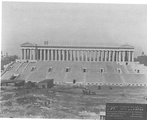
Figure 3. Completed west colonnade, 1924 (Chicago Park District Special Collections)
