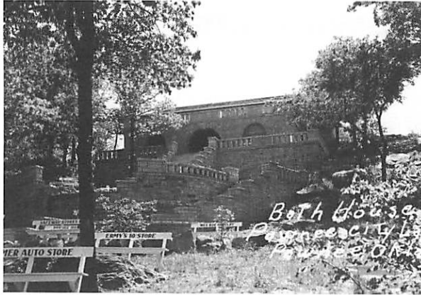
Figure 1. Bathhouse, 1940 (City of Pawnee)
