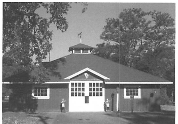
Figure 2. Stud Barn, circa 2004. The stud barn built by Charles Howard especially for Seabiscuit was the racehorse's home from 1939 to 1947. The barn, currently being restored, serves as the centerpiece of the preservation project for the Howard-era buildings. (Seabiscuit Heritage Foundation)
