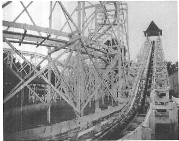
Figure 3. An early wooden roller coaster, Leap the Dips in Altoona, Pennsylvania, is still a central attraction at Lakemont Park (Photograph by Tom Halterman, National Register collection)
