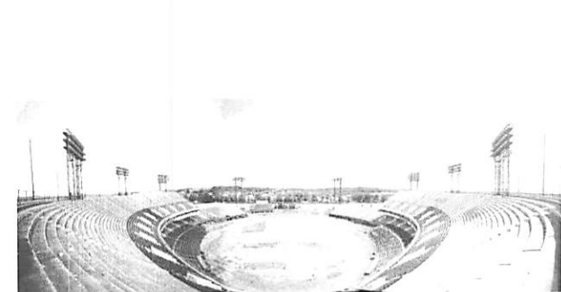
Figure 10. Baltimore's multipurpose Memorial Stadium (1953) was once called "the world's largest outdoor insane asylum." It was replaced by two separate stadiums for baseball and football in the 1990s. Photographs by James Rosenthal, 2000, prior to demolition; panorama stitched by Charu Chaudhry.
