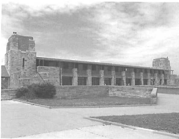
Figure 7. View of the East Bathhouse south facade, 2004. This is one of many photographs of Jones Beach taken for the SPLIA report from the vantage point of an historic original (refer to figure 1). When compared, the two images tell a compelling before and after story. In this image, the clock face is gone, the landscape is bare, and canvas awning and wooden support members are replaced by aluminum and fiberglass. (A. Parsons Wolfe)
