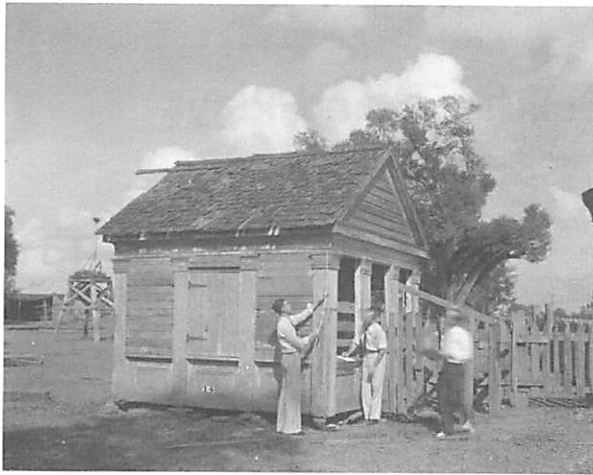
Figure 1. HABS team measuring Angelina Plantation Doll House (circa 1840) in Louisiana in 1934. Photograph by Paul Koch. HABS/HAER/HALS continues to employ student interns to do complete fieldwork on project sites around the country. (All illustrations from the HABS/HAER/HALS collection)
