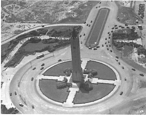
Figure 4. Aerial view of the Water Tower looking west, showing an oval-shaped reflecting pool at the Ocean Parkway median and traffic flow around the turning circle, 1938. A pedestrian pathway is also visible running under the reflecting pool of ocean Parkway. (Long Island Region Photographic Archive, New York State Office of Parks, Recreation and Historic Preservation)
