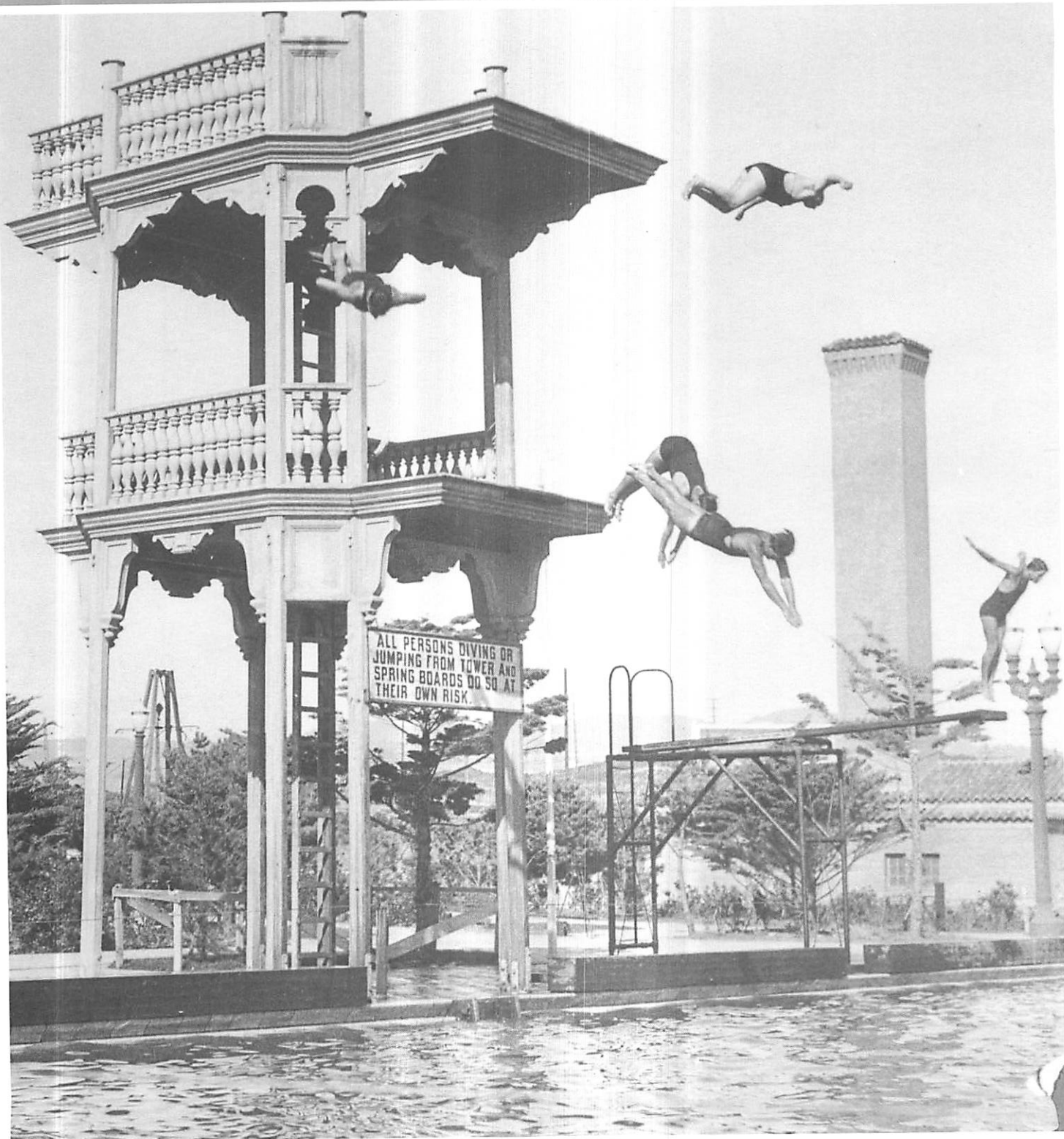
Fleishhacker Pool, constructed 1925, San Francisco, California (HABS photograph from San Francisco Room, San Francisco Library, Civic Center)
