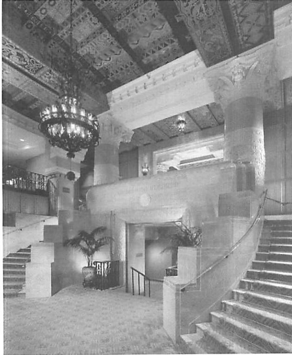
Figure 10. Historically the symmetrically designed two story lobby at the MAC featured a double set of marble stairs curving up to the mezzanine, with buttress steeped side walls of marble, and brass hand rails. At the top of stairs were thick marble and terra cotta columns with capitals featuring lotus leaves and warrior heads. (NPS file)
