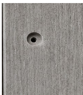
1.A Pre-Drilling and Countersinking
