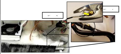
d. IMPORTANT: Do not install the Thermistor over the ridge at the tubing seam (See
