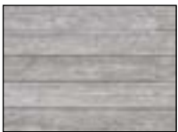
Board Formed Concrete
