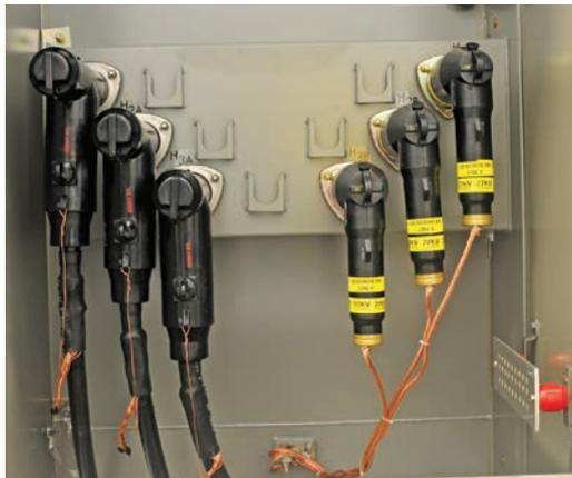
**Figure 6** The high-voltage side of distribution transformers specified with dead-front construction uses elbow connectors. The surge elbows on the right integrate MOVs to provide overvoltage protection.
