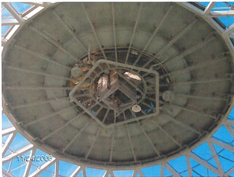
Figure 7: Underside of Show Dome Apex
